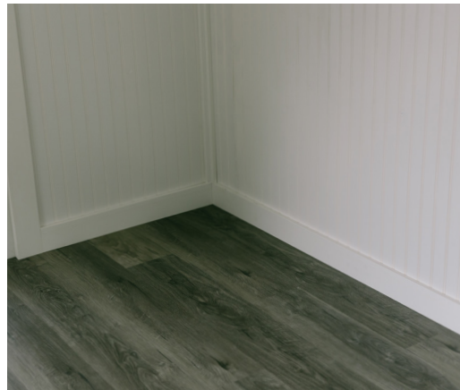
Vinyl plank interior flooring
