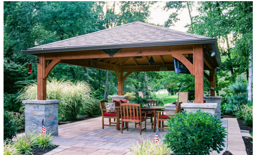
Hip style, wood material, shingled roof, standard beam, exposed rafters
