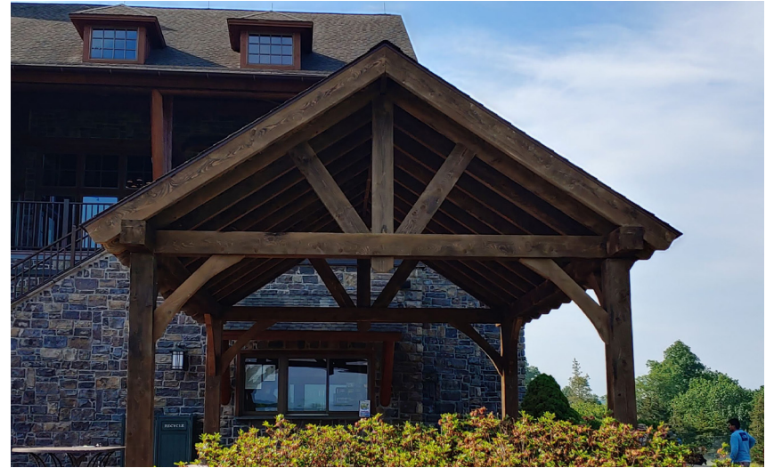
Open gable A-frame style, stained wood material, shingled roof
